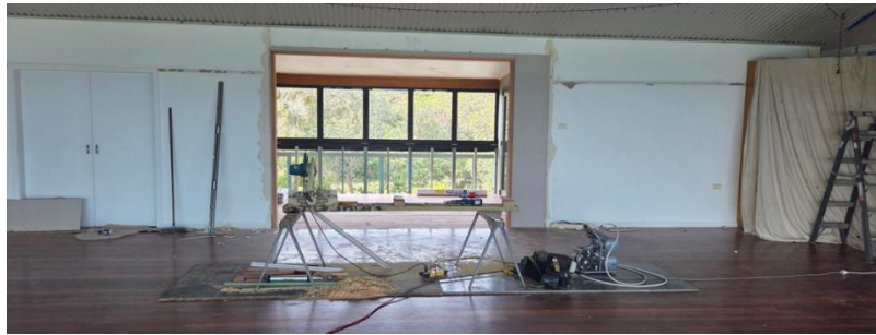
Enclosing the deck (2025)
