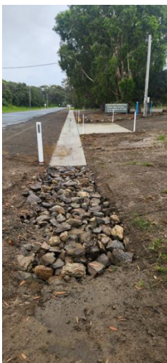
Street dish drain (2024)
