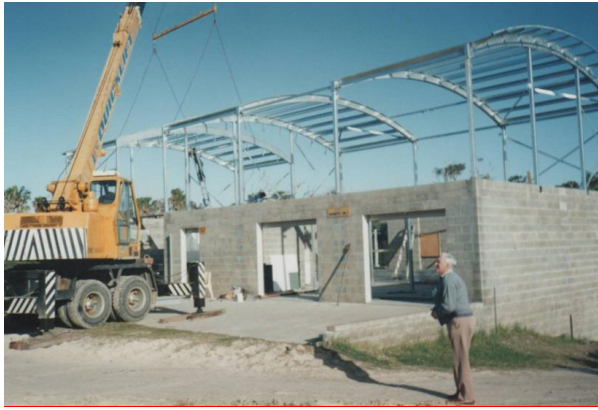
Stage 4 construction Aug 1993
