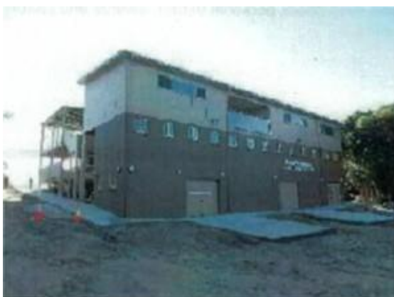
Recently constructed pathways
