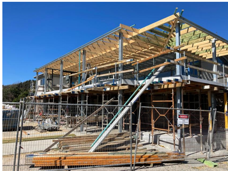
Stage 6 Deck and storage
