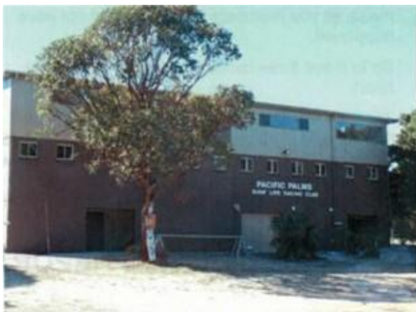
New extensions almost complete.
