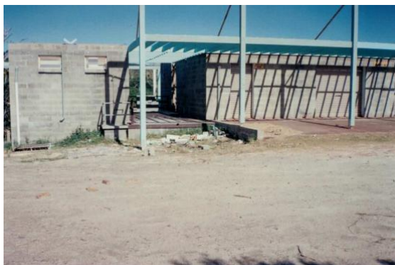
Building works July 1993
