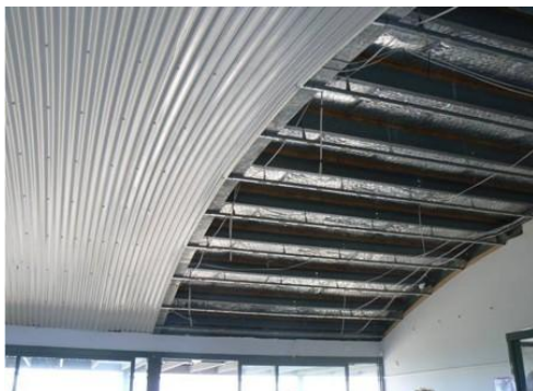
New acoustic ceiling
