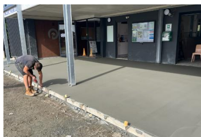
Concrete slab replacement (2026)
